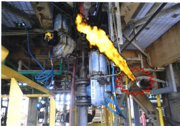
The flame affected to radioactive source of 08C108.
